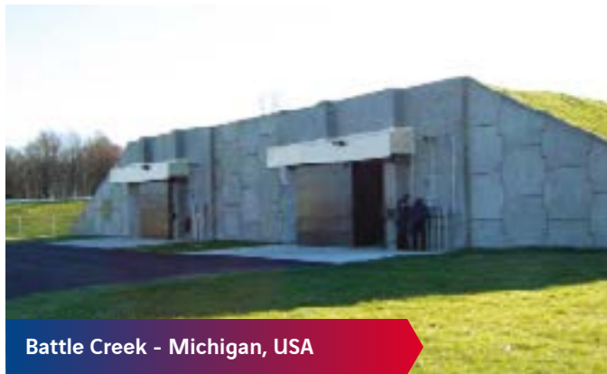
Magazine, Precast Concrete Earth Covered - USA
