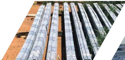
Steel strips reinforcement
