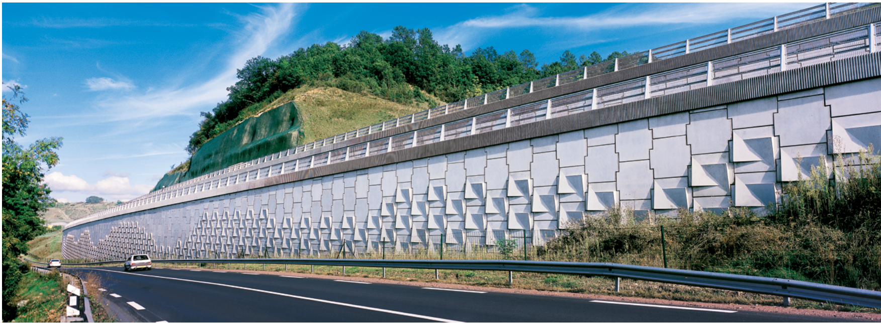
Motorway A89 from Saint-Astier to Arc 2.3 ◀ Mussidan-Périgueux, France
