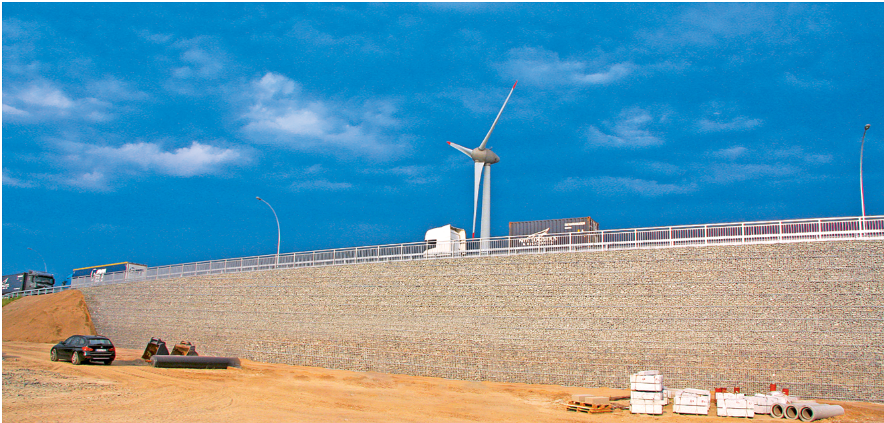
Retaining Walls in Altenwerder
