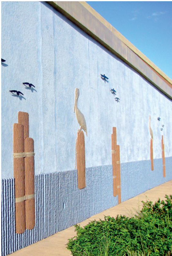
State Highway SH-358 at Weber Road Corpus Christi, Texas, USA ▶
