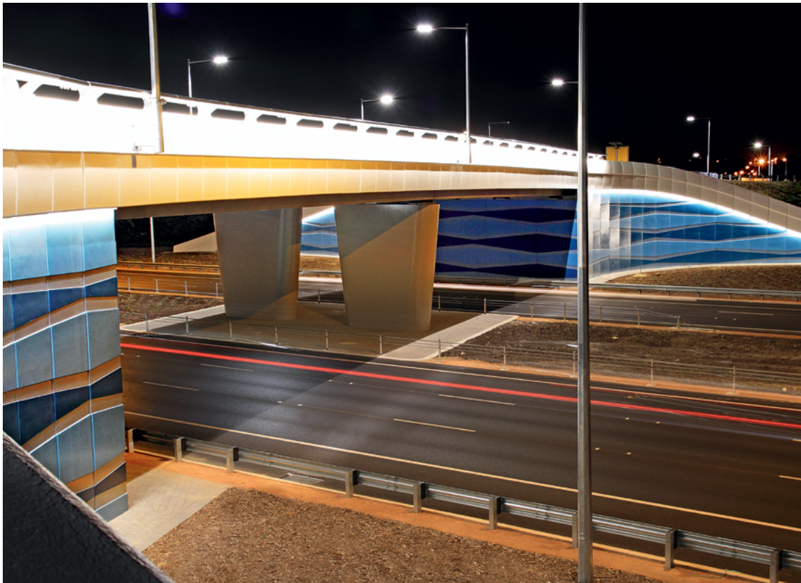
Tonkin Highway / Dunreath Drive Interchange, Gateway Western Australia Perth, Western Australia, Australia ▶
