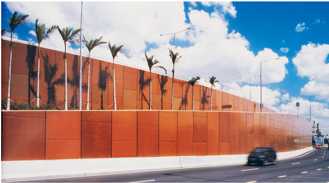
Inner City Bypass Brisbane, Queensland, Australia ▶
