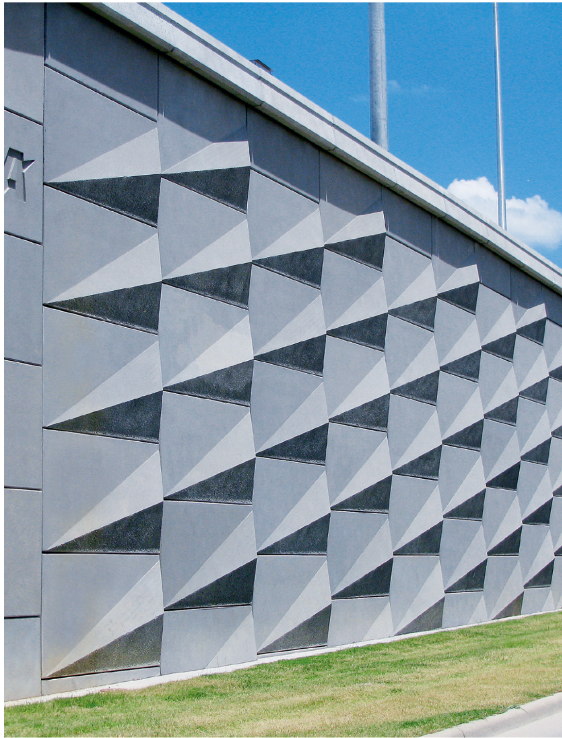
Sam Rayburn Tollway at Lake Forest Drive ◀ McKinney, Texas, USA
